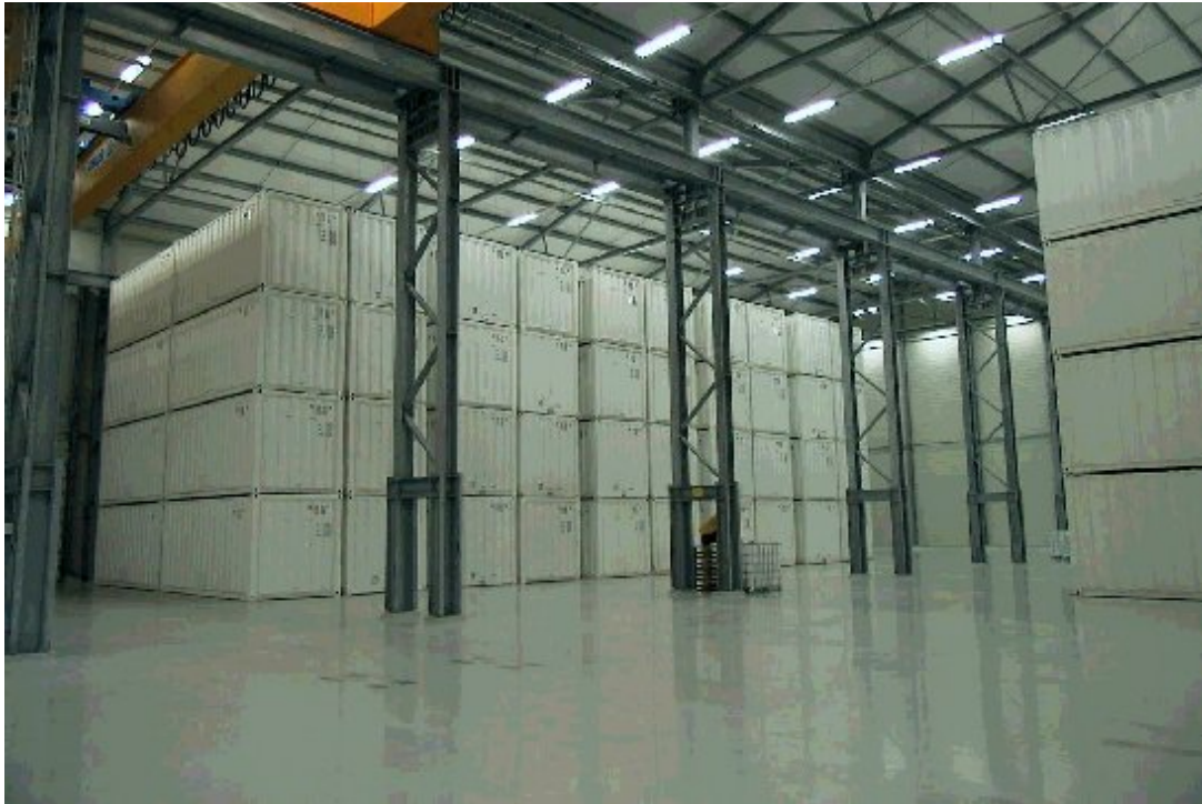
Figure A.3. The storage of radioactive calcinate from phosphor production
