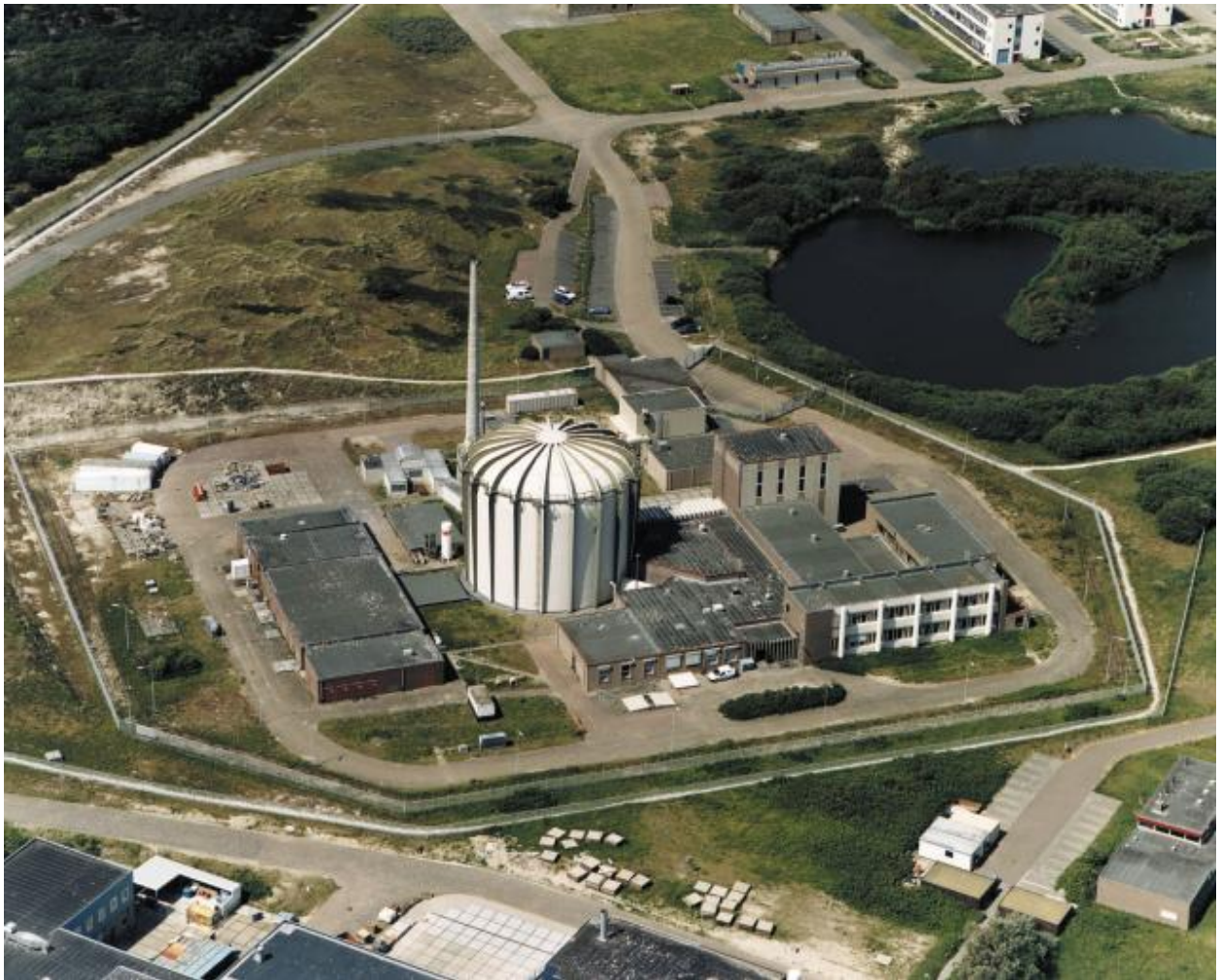
Figure 1-4: Aerial photograph of the HFR site
