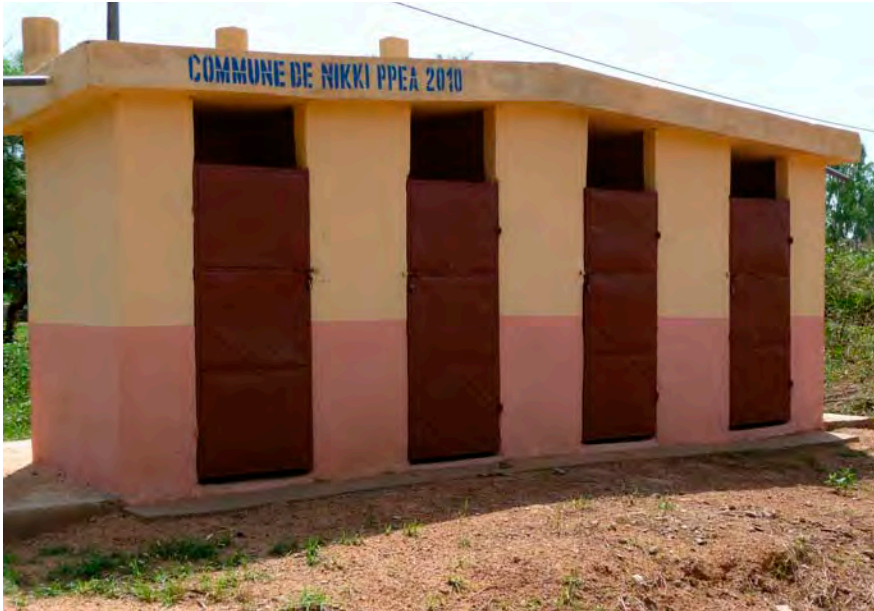
Latrines in institution
