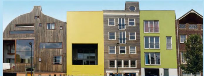
3 Modern buildings inspired by Dutch canal houses from the 17th century, IJburg, Amsterdam (p. 12-13)
