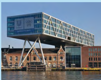
7 Headquarters of Unilever on the Maas river, Rotterdam (p. 22-23)
