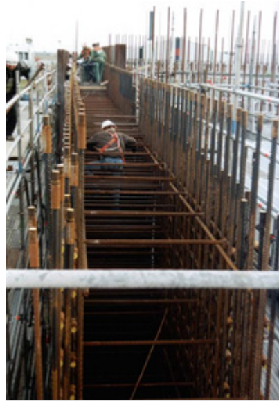
Figure A.5. Worker in the concrete at work in a 1.7 meter thick outer wall
