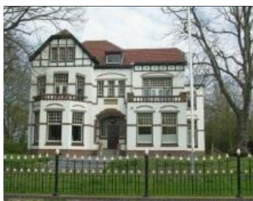
Figure 5.8 Examples of some of the typical unreinforced masonry building typologies found in the Groningen region
