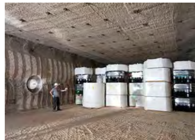
Figure 2-6: The WIPP facility in bedded salt formation in New Mexico, USA, for the disposal of defence transuranic and other wastes. This cavern has been excavated in the salt using conventional mining techniques.
