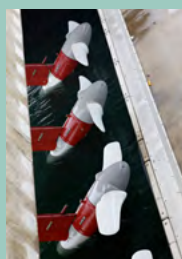
Water turbines in the Oosterschelde barrier are used to induce energy from changing tides (p 20)
