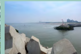
Innovative ways to reinforce dikes and sea barriers near Cadzand (p 33)
