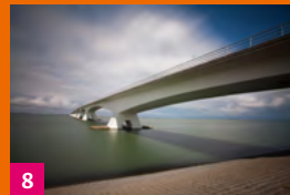
8 The Zeeland bridge. (p 14)
