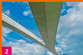
2 The Nescio bridge over the Amsterdam-Rijnkanaal, one of the longest bicycle and pedestrian bridges of the Netherlands. (p 5)
