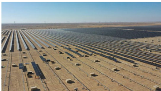
The Ibra II 500-megawatt photovoltaic independent solar power plant in Oman. Once finished, the plant will cover 13 square kilometers. Photo © AIIB 2021
