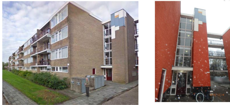
Figure A.33 Side view (left, from Google street view, in 2009) and particular of the entrance (right, left, from [Arup 2017d], in 2014) of Abel Eppenstraat 15-69.
