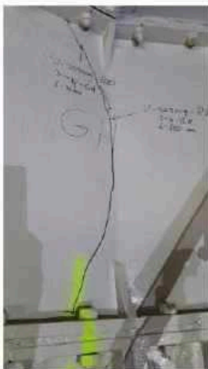
Door-en-door verticale scheur wandpaneel (ref. 1,2021)
