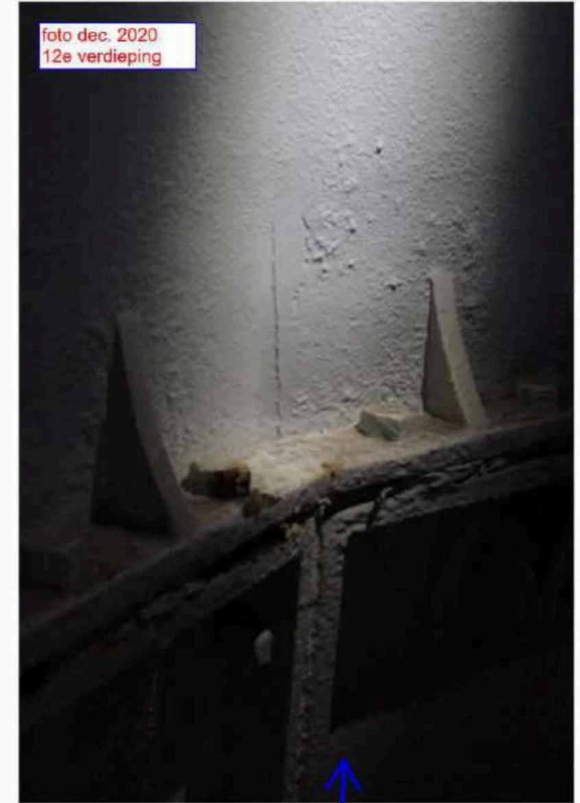
Verticale scheur in wand
