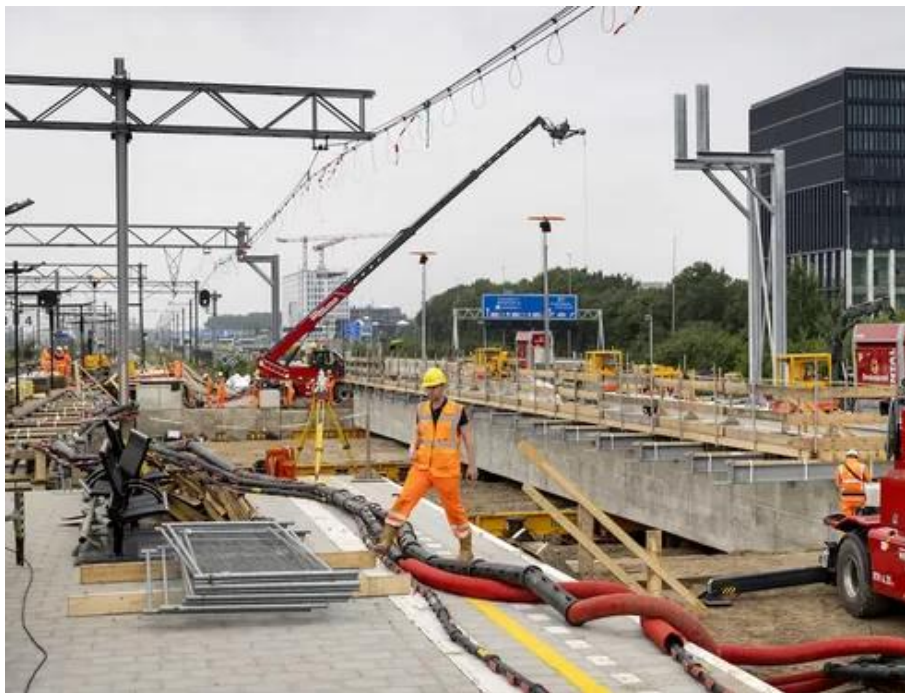
Dakdelen Brittenpassage Station Amsterdam-Zuid
