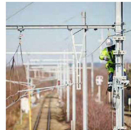
Electrification works between Genk-Goederen and Bilzen (L21C)
