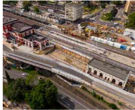
Lugano-Besso underpass construction site.
