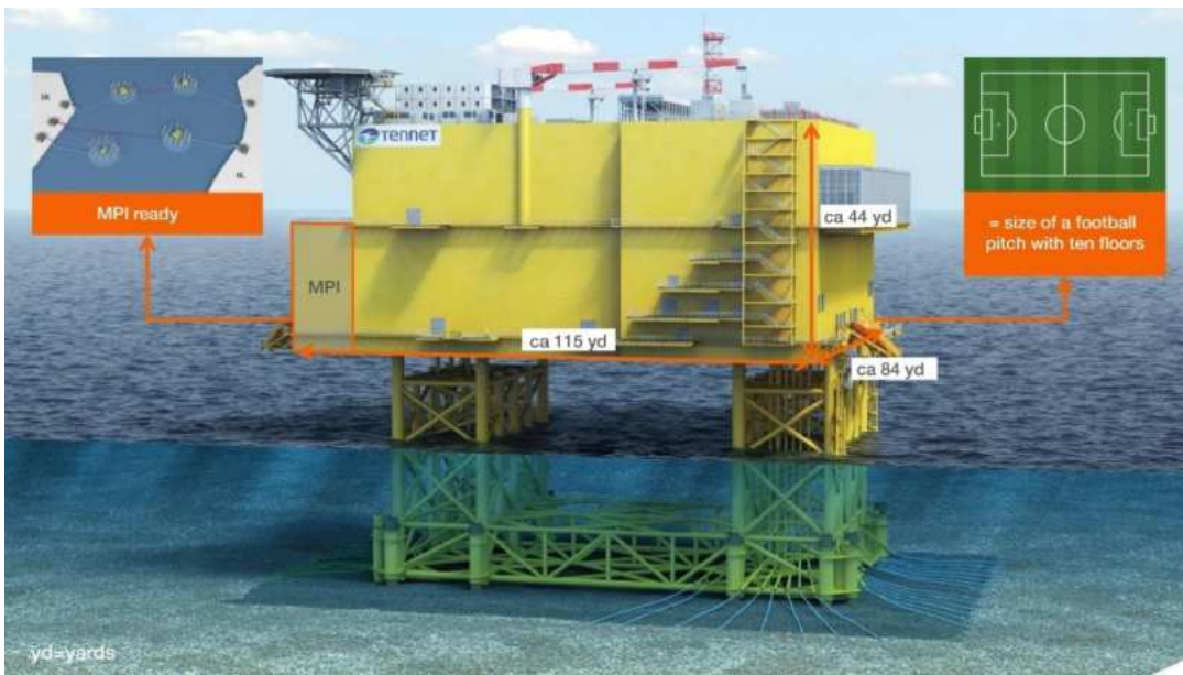
Figure 6.18: Standard 2GW HVDC platform (ref. 44).
