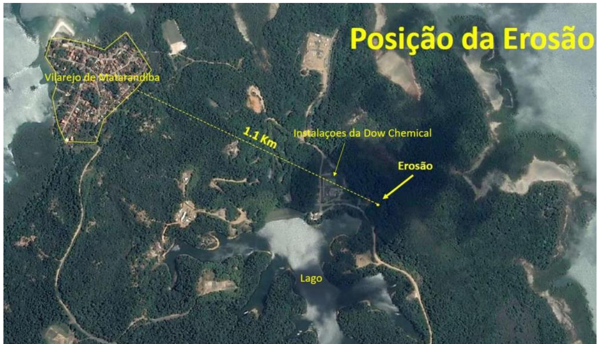
Figure 88. Sinkhole location in Matarandiba Island (from G1, 2018).
