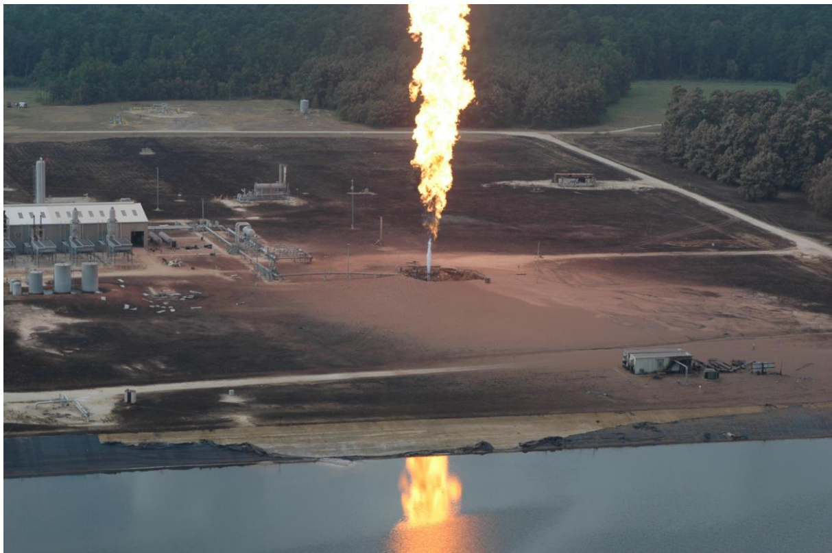
Figure 41. Blowout and fire at Moss Bluff.
