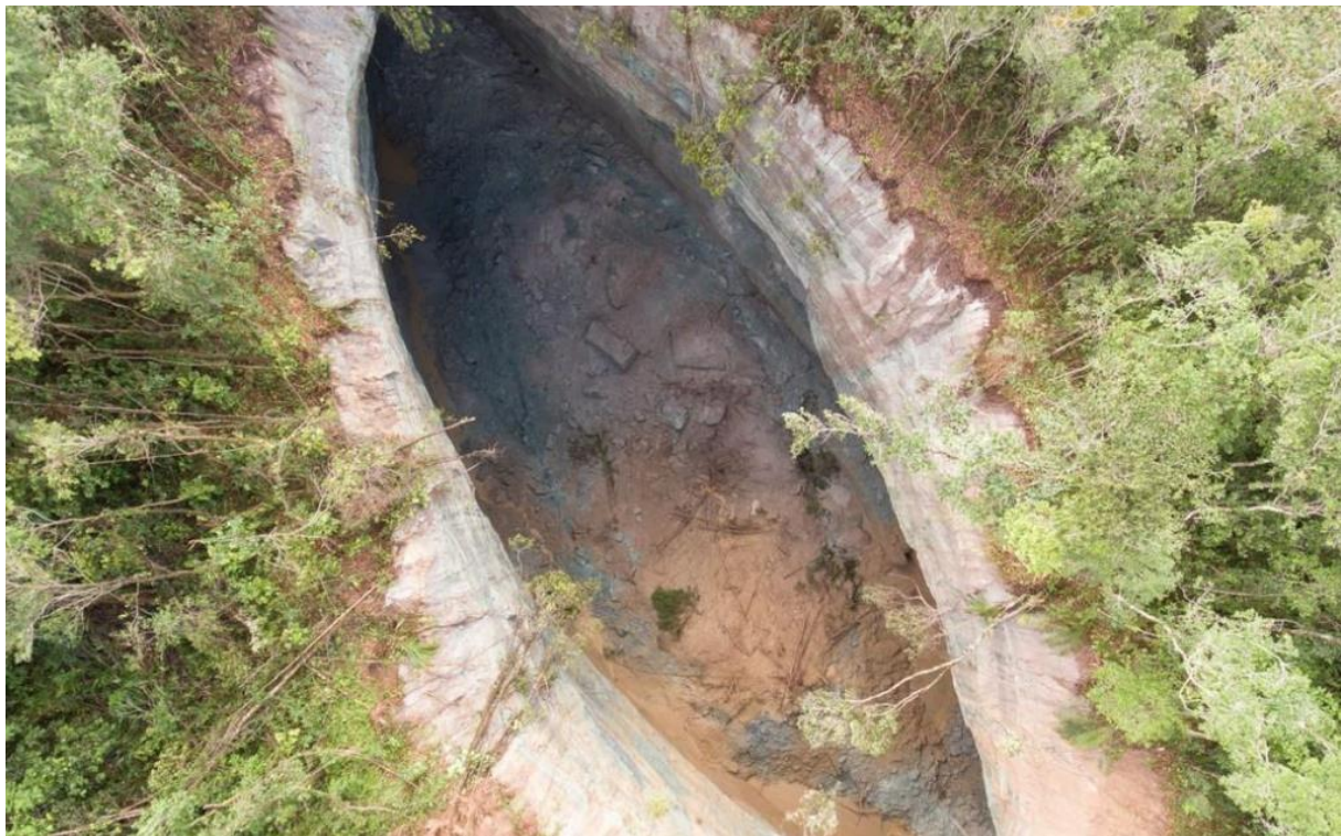
Figure 89. Drone view of the sinkhole location in Matarandiba Island (from G1, 2018).
