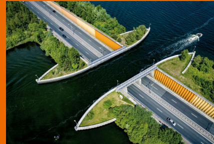
This navigable aquaduct allows boats up to 3 meters deep to pass into the Veluwe Lake, allowing road and naval traffic to coexist.
